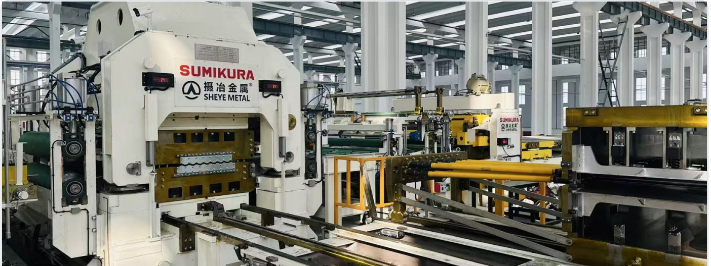
INTERCHANGEABLE LEVELLING CASSETTE SYSTEM ON THE SUMIKURA LINE
