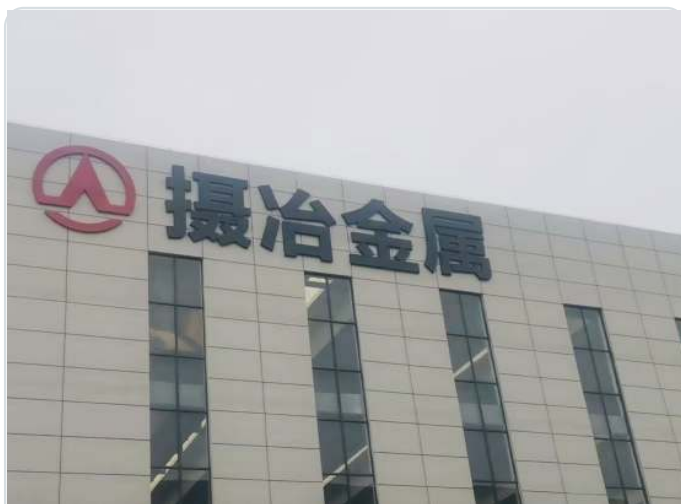
LIYANG HIGH-END COIL AND SHEET CENTER
